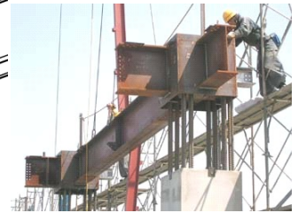
Erection of beam and joint as a unit
